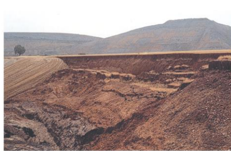
Figure 9.12 Curved failure in clays and shales in central Spain, showing the tension crack and vertical displacement of the slope head.
