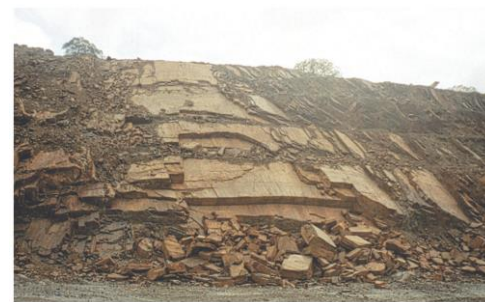
Figure 9.17 Plane failures along bedding planes on slope benches (slope height: 60 m).
