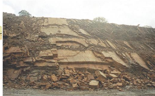
Figure 9.17 Plane failures along bedding planes on slope benches (slope height: 60 m).
