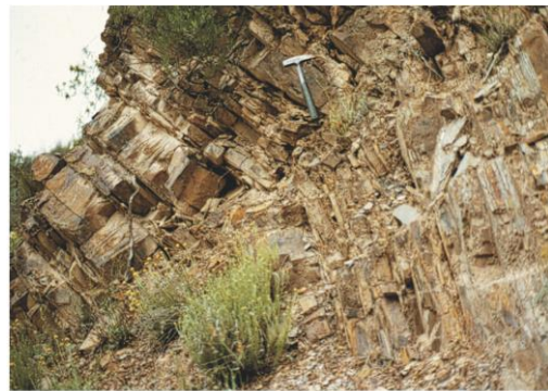
Figure 9.22 Rock blocks on a slope where toppling has occurred.
