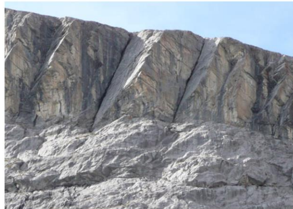
Fig. 8 Scars of wedge failures in limestone, Canmore, Alberta, Canada. The cliff is approximately 50 m high (Photo by O. Hungr)
