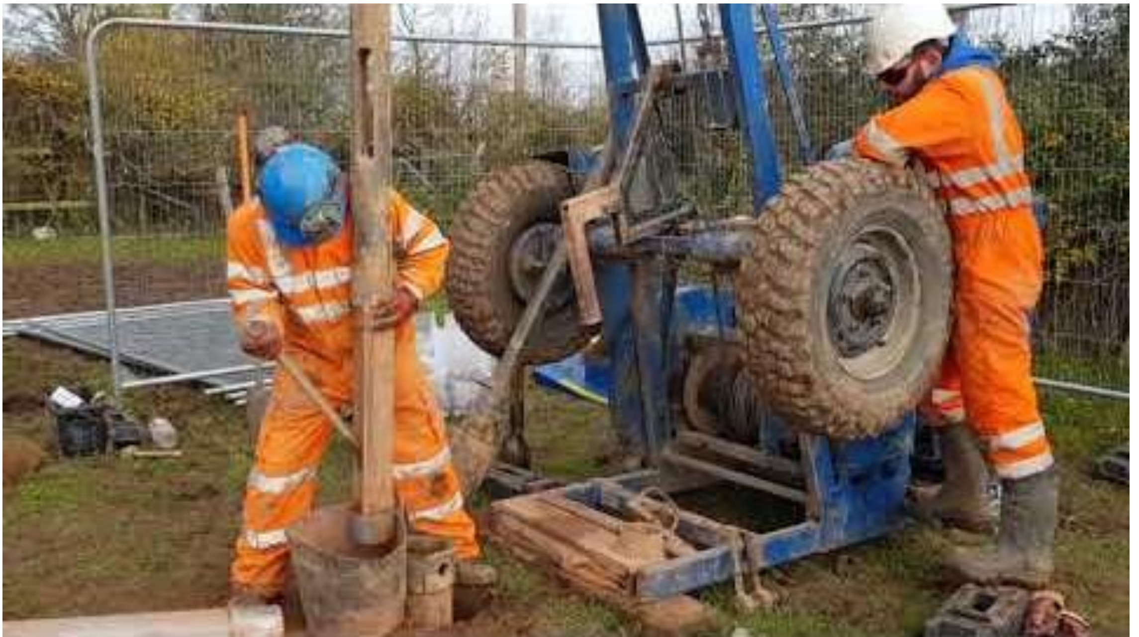
衝鑽法 Cable Percussion Boring
