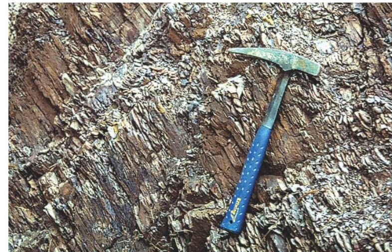
Palaeozoic slate. Very poor quality. Heavily jointed. Degree of weathering: V.
